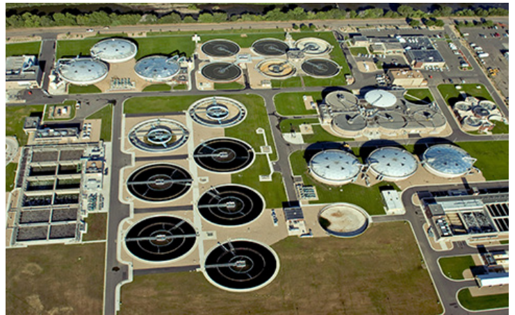
The plant's large size and sprawling layout created a challenging environment for manual data collection. Automated data collection has resulted in time savings and greater data accuracy and reliability.
