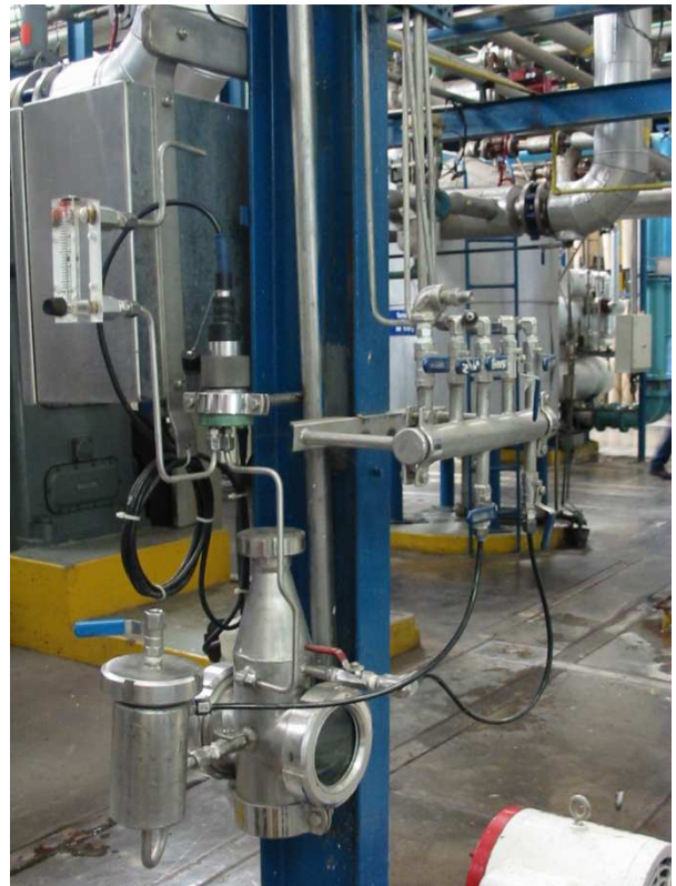
Fig. 4 Another configuration of CO 2 sampling
